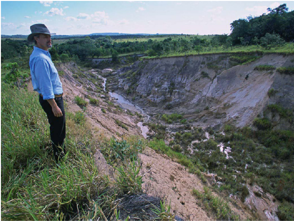
Erosion in Brazil after 10 years of production in the Cerrado
